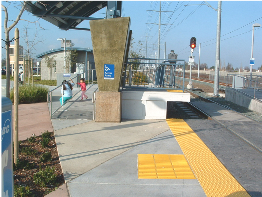
PLATE C-7: MINI-HIGH ACCESSIBLE RAMP
