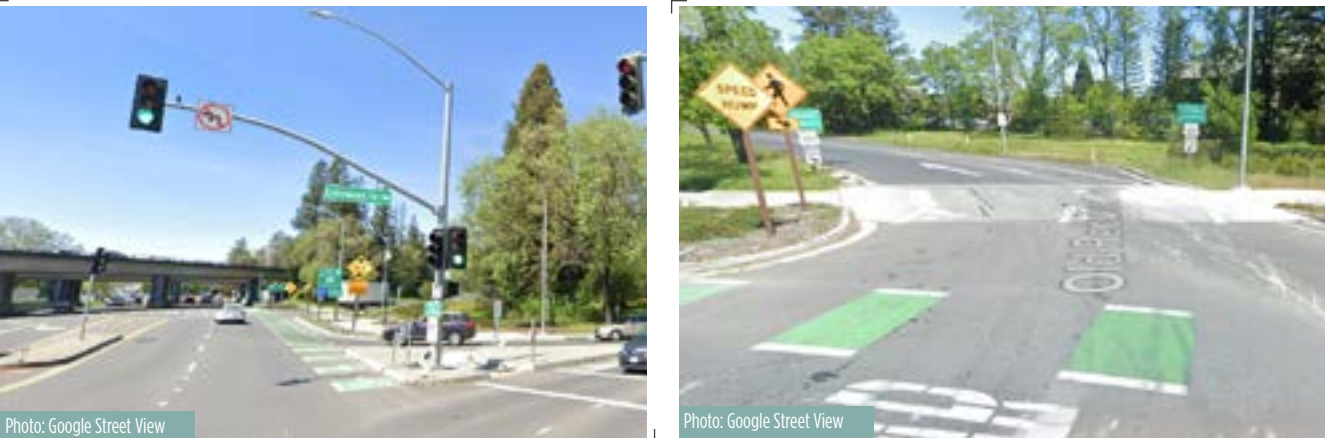
The US 101 ramps in Windsor, CA include green bike lanes, compact design, and a raised crosswalk across the on-ramp.
